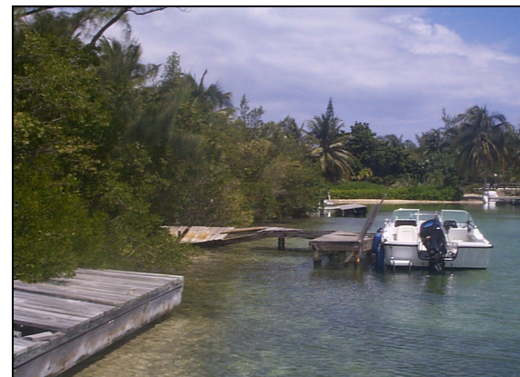
Photo 3: Enforcement action may result if a dock is not maintained to a safe standard or if the damaged dock is impacting the natural environment.
