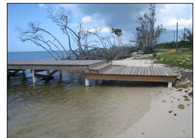
Photo 1: Good example of a dock design which does not block pedestrian access between the low and high water marks.
