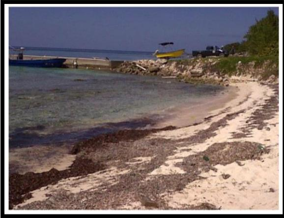
Figure 2: Showing coastal erosion to the east of the dock in 2011 one year after dock is rectified and poured solid with concrete (Source: Ministry of DATT, January 2020)
